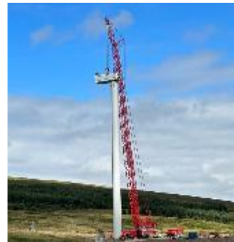
Capital Dynamics Pines Burn site during construction
